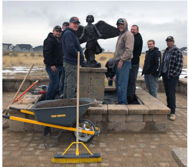
Teamwork: setting the statue on its foundation
