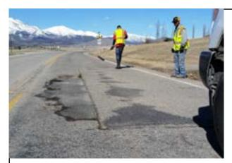
The common method used to treat them has been to send out a crew with asphalt and fill the holes. The problem with this is the same reason we don't build roads in the winter - it doesn't work very well in winter conditions. This method is better than nothing but often needs to be repeated until the weather warms.
