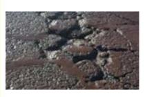
is why crack sealing is part of our annual maintenance. Potholes form when water works its way down into the road material and temperatures drop below freezing. The freezing water expands and causes a swell. When the tar that holds the road together freezes it becomes
