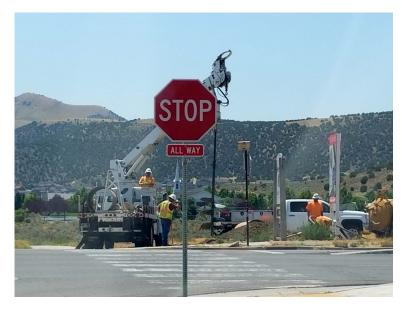
Some construction activity is underway at Pony Express Parkway and Porter's Crossing. Prep work is being done for the future traffic signal at that intersection. Poles are expected to be placed in October.
