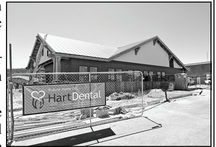
The future home of Hart Dental — under construction in The Ranches.
