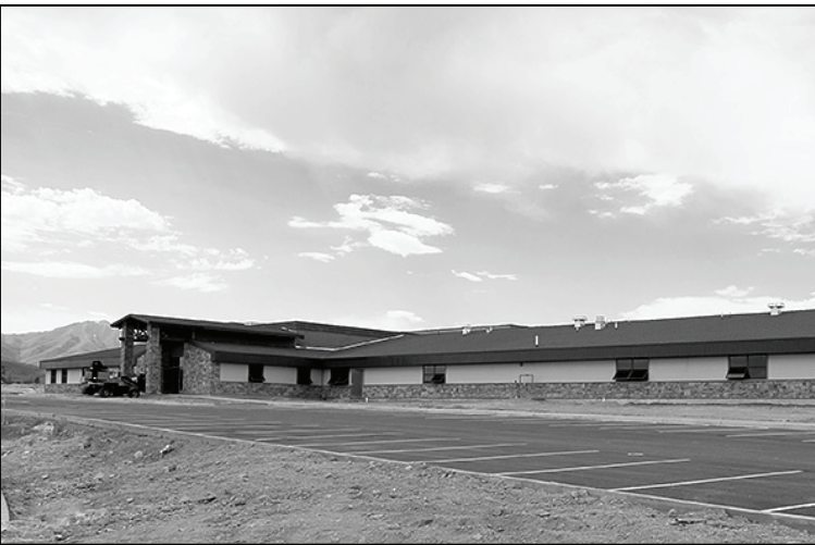
Rockwell Charter High School is 62,000 square feet, with a high school wing for grades 10-12 and a junior high wing for grades 7-9.
