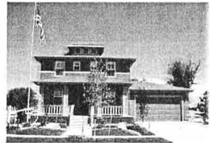
This image shows the siding elevation of the same house: it's EA Ratio is 0.57.
