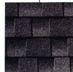
ROOFING Material: Asphalt Shingles Color: Moire Black
